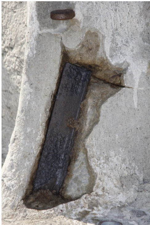
Figure 9: repair removed, metal treated
