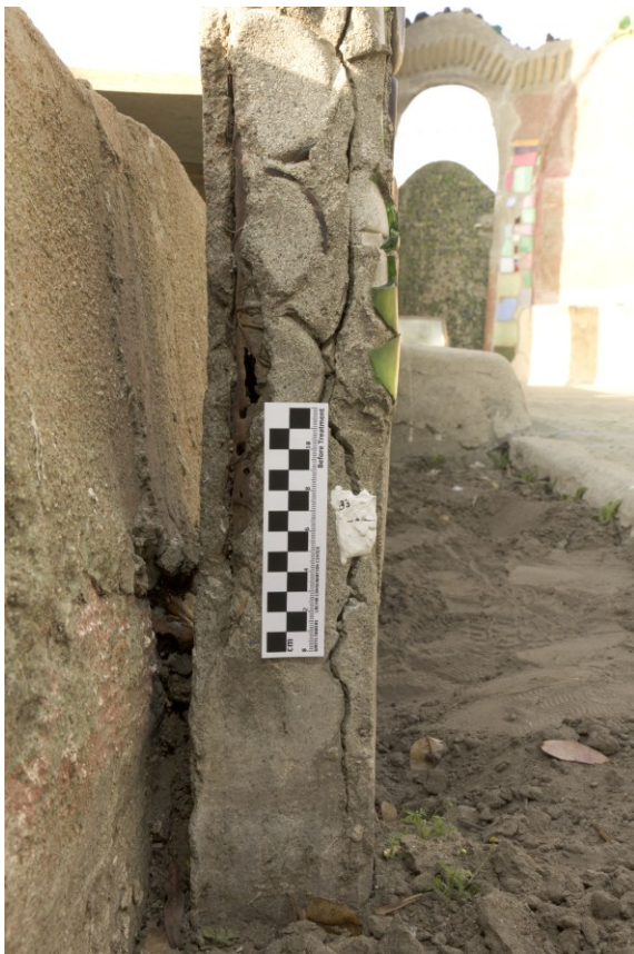
Figure 15: Before pinning
