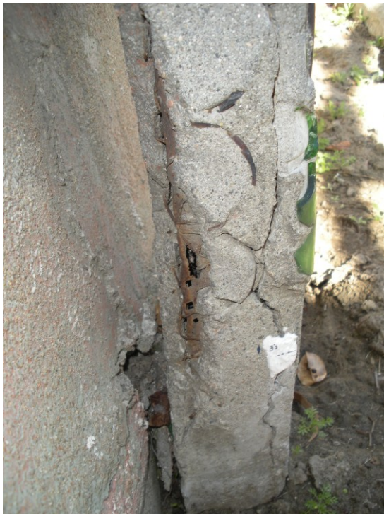
Figure 13: Post 5, pre-treatment condition
