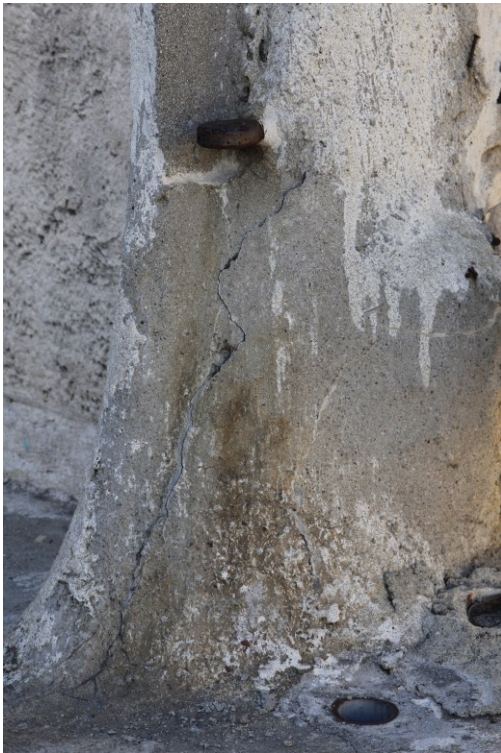
Figure 7: Cracked and detached repair at garage
