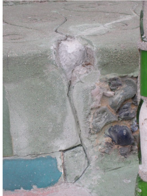
Figure 12: WTO base after removal of repair
