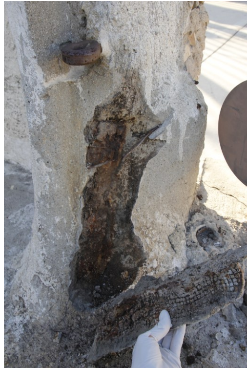
Figure 8: During removal of old repair
