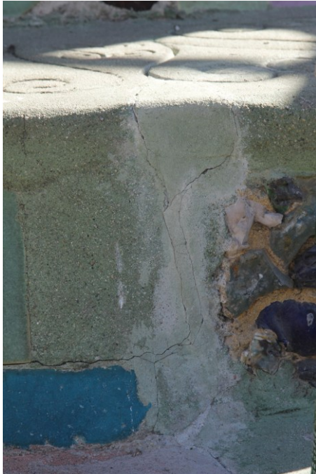
Figure 11: WTO base, 2001 & 2005 repairs
