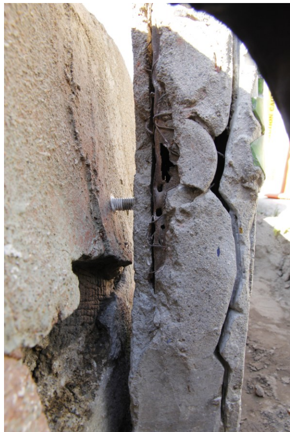
Figure 16: After pinning
