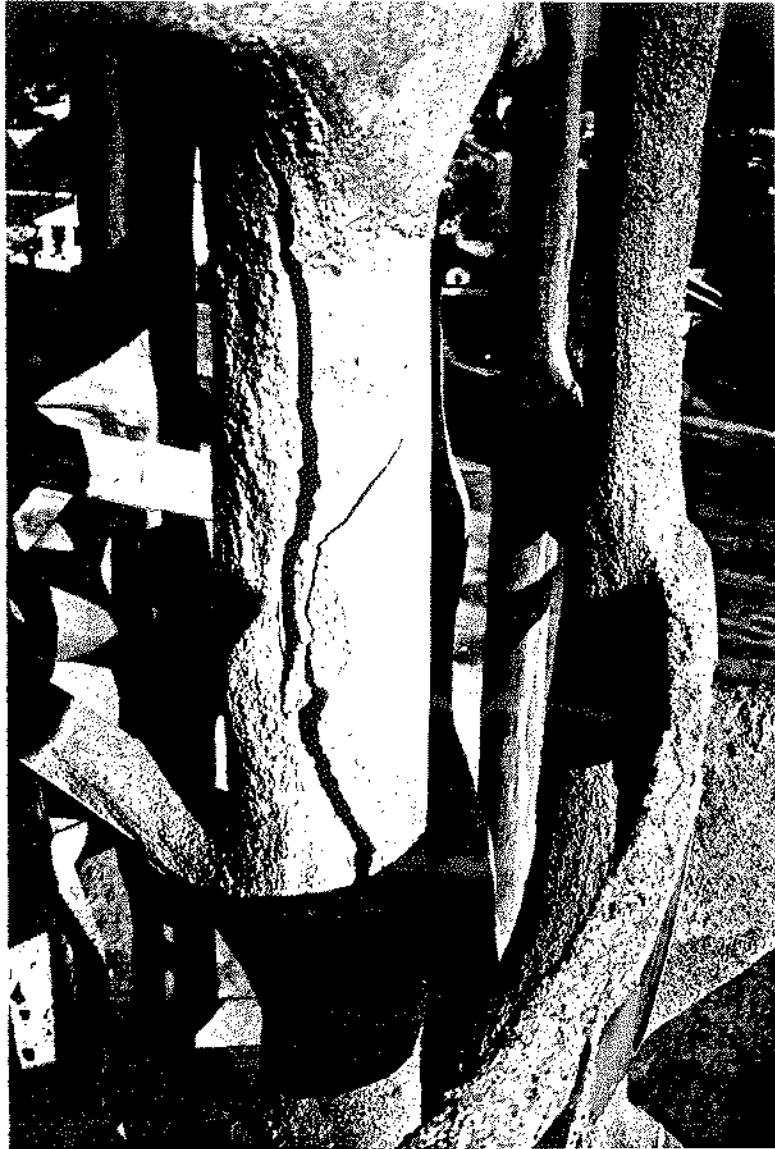
Photograph 46. Crack in Center Tower vertical column before repair from boom bucket. December 16, 1992 Figure 36.
