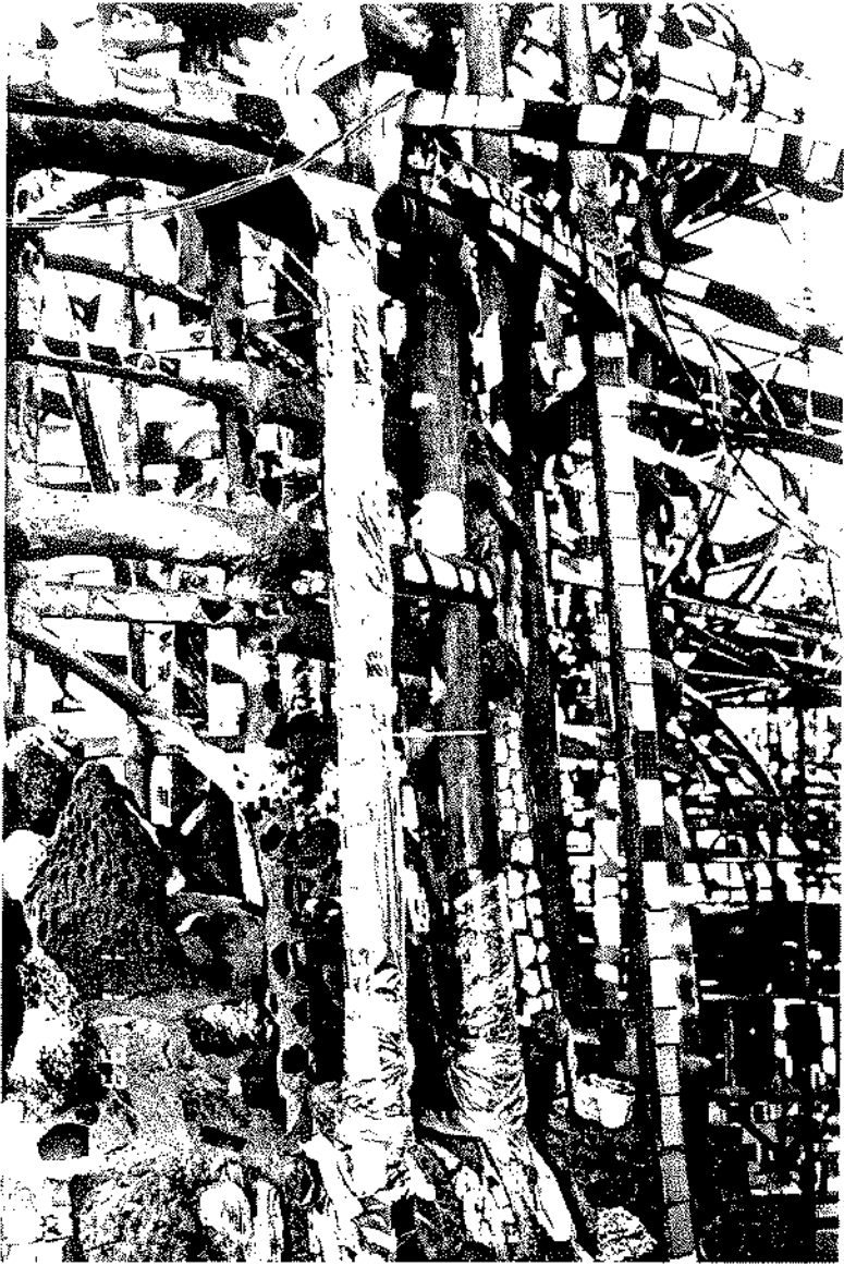
Figure 10. Center Tower showing some of nine support columns wrapped with plastic to impede rain water intrusion into large cracks in mortar. 1/11/93 photo.
