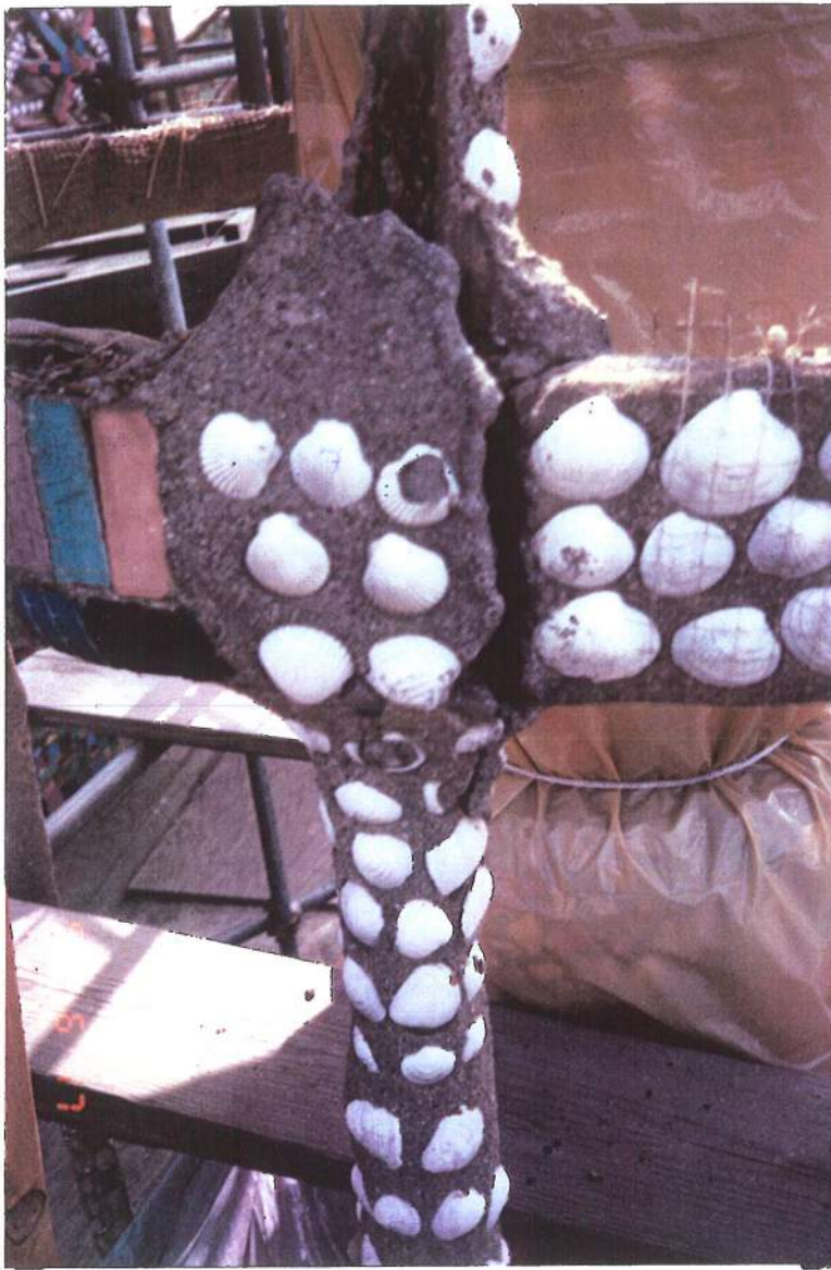
Figure 9. Major crack at Band-to-vertical joint. Jun 1991. ATO C W.
