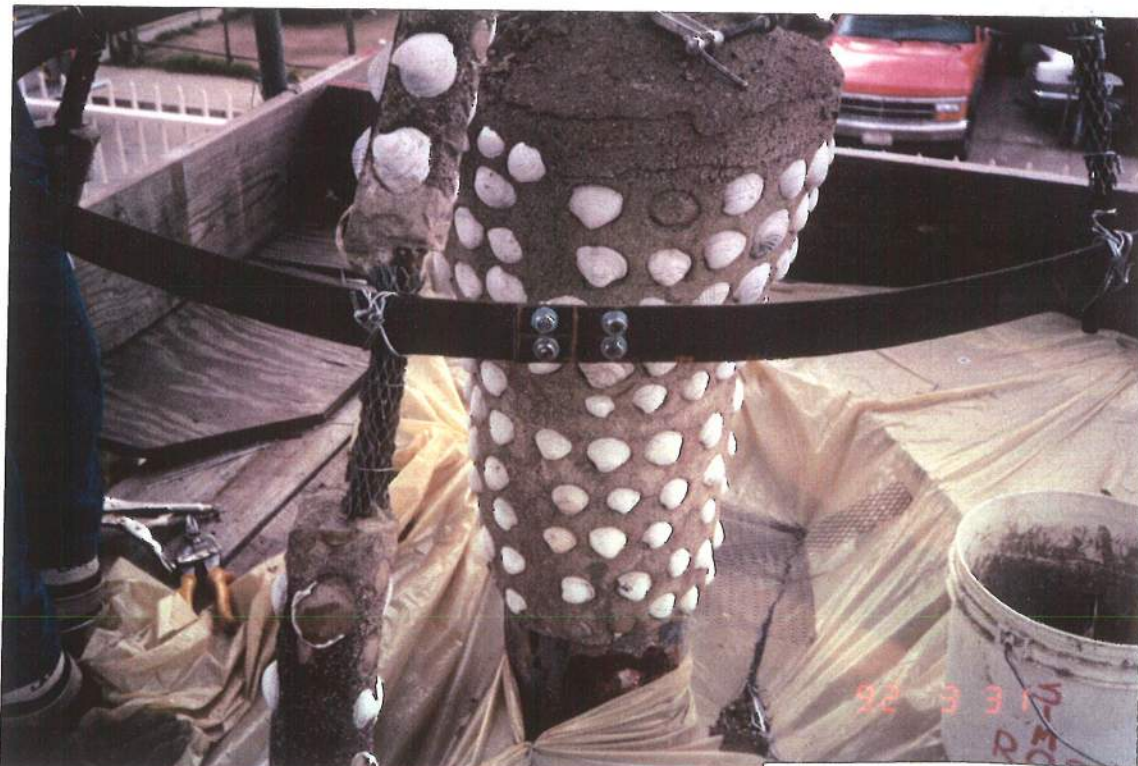
Figure 37. Attachment of new steel for Maj Band 03 before rebonding of original mortar. March 1992. ATO C N.
