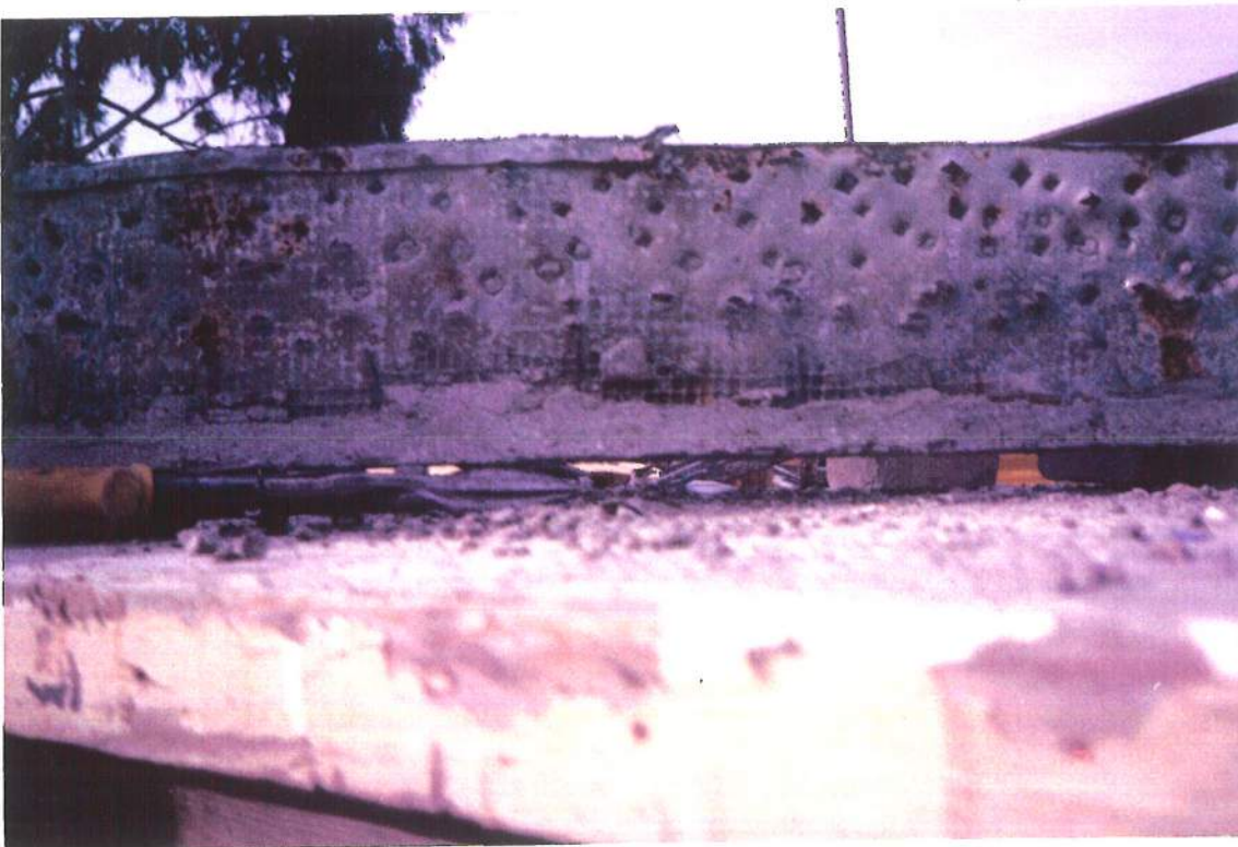
Figure 31. Damaged sheet metal rebar detail from Maj Band 01. Dec 1991. ATO B N.
