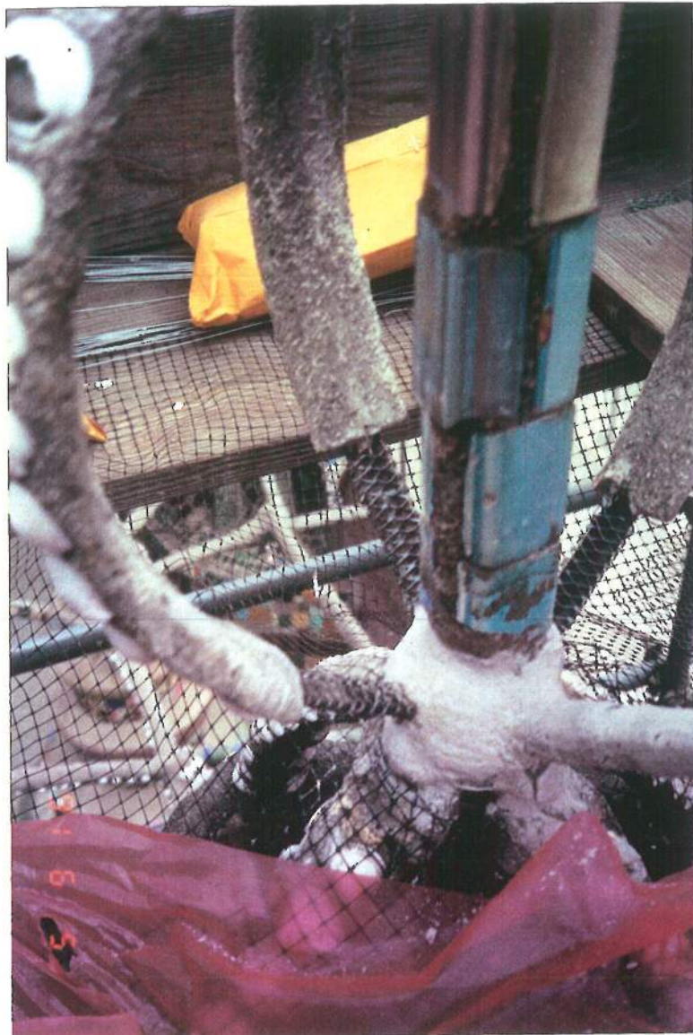
Figure 26. Detail showing mortar build-up to original contour. Jun 1991. ATO SE E.
