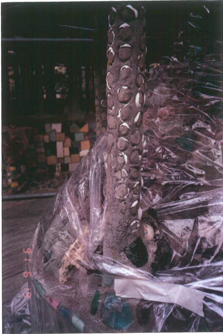
Figure 16. Major vertical 04 before removal of damaged mortar and replace- ment of steel reinforcement. Jun 1991. ATO B W.
