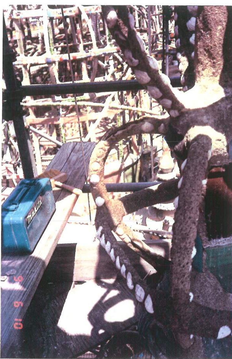
Figure 5. Damage to top of major vertical no. 04, top center of photo. Jun 1991. ATO D NW.
