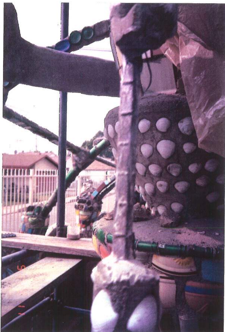
Figure 29. Rodia rebar major vert- ical 02 exposed for cleaning and repair of mortar at Maj Band 01. Dec 1991. ATO B E.
