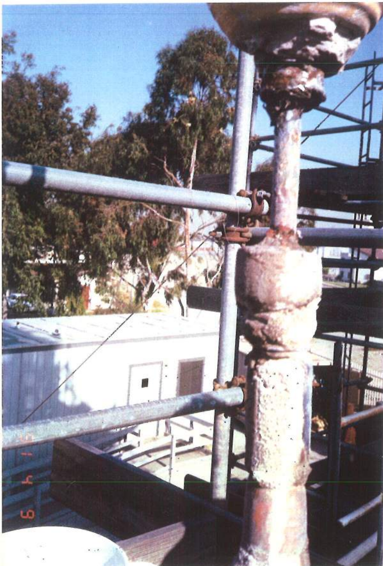
Figure 4. Steel rebar uncovered near top of spire on "A" Tower. Apr 91. ATO E SE.
