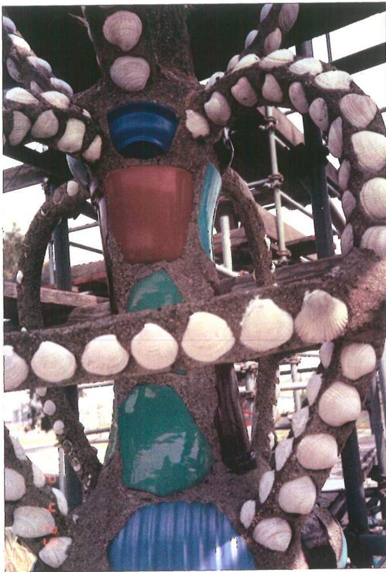
Figure 38. Ornaments after clean- ing & consolidating with DF-104/B-72. April 1992. ATO D SE.
