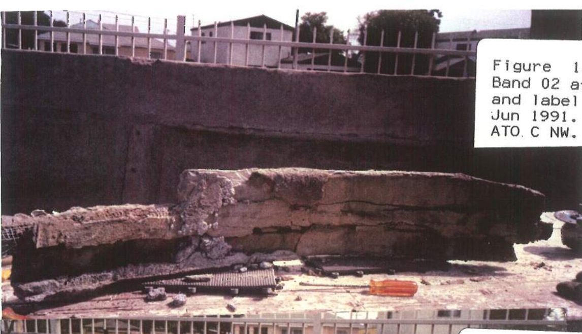
Figure 14. Band 02 portion on bench after removal for repair and replace- ment of reinforcement. Jun 1991. ATO C NW.
