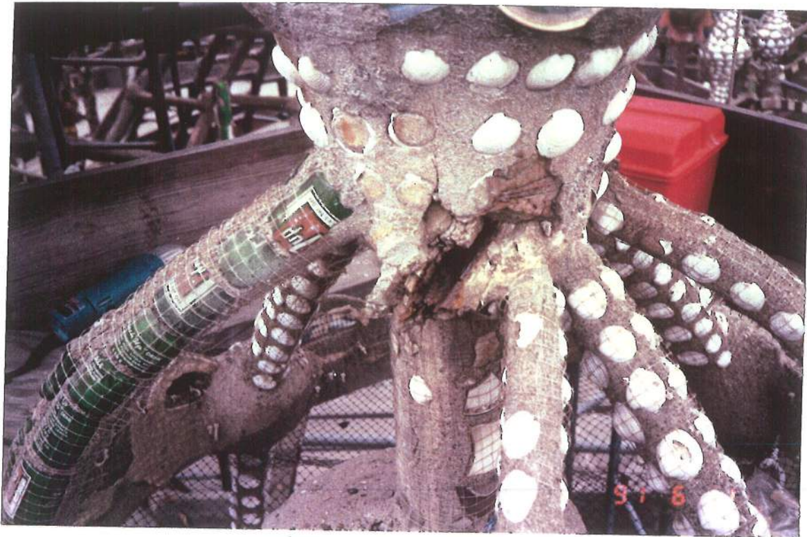
Figure 28. Top joint after removal of major vertical 04 for replacement. Jun 1991. ATO D SW.
