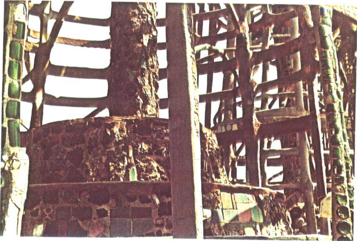
PHOTOGRAPH #12 EXISTING HORIZONTAL CRACKS WIDENED BY EARTHQUAKE DAMAGE 10/04 TO WEST TOWER COLUMN
