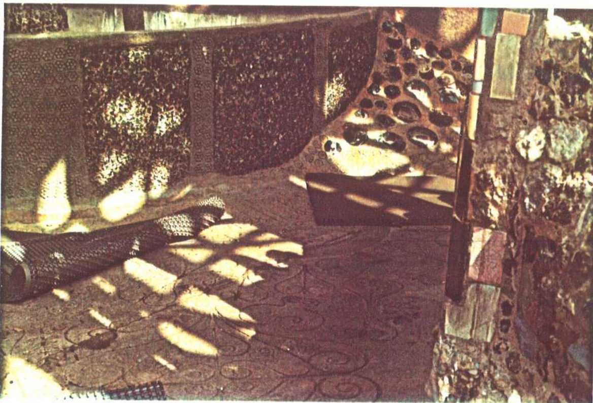
PHOTOGRAPH #04 EARTHQUAKE DAMAGE 10/04 TO PATIO FLOOR BETWEEN CENTER AND WEST TOWERS PHOTOS BY N.J. GOLDSTONE
