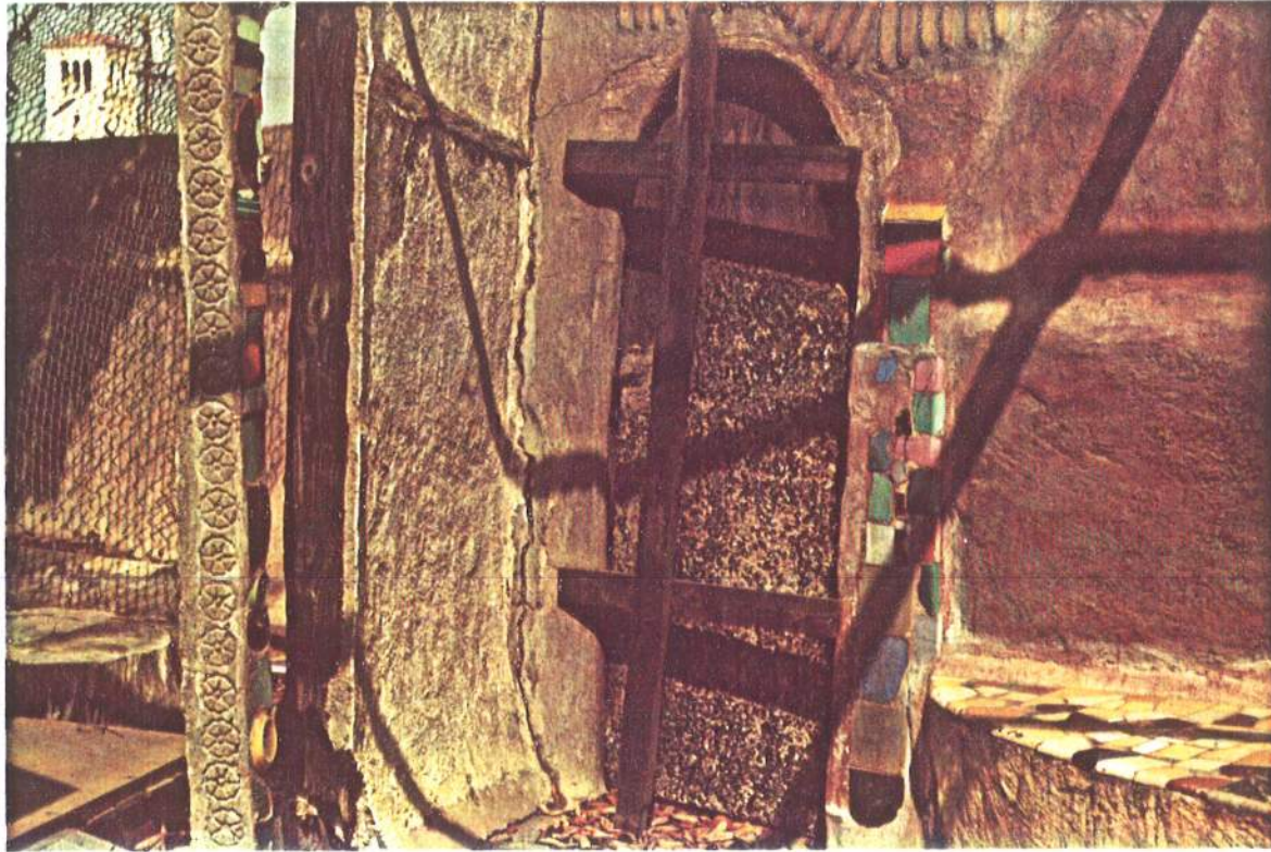
PHOTOGRAPH #06 EARTHQUAKE DAMAGE 10/04 TO VERTICAL JOINT BETWEEN NORTH WALL AND RODIA HOUSE FACADE
