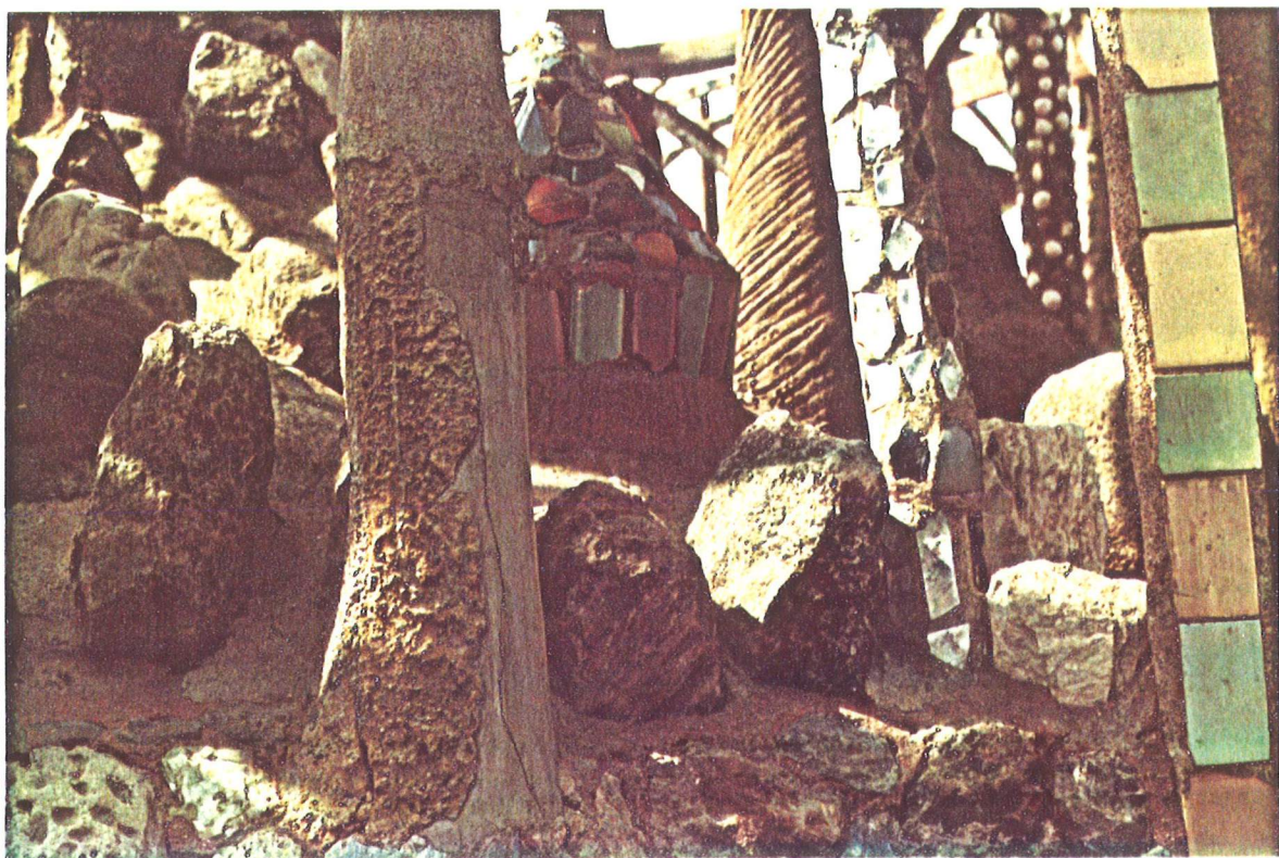
PHOTOGRAPH #11 EXISTING CRACK WIDENED BY EARTHQUAKE DAMAGE 10/04 TO CENTER TOWER COLUMN #8
