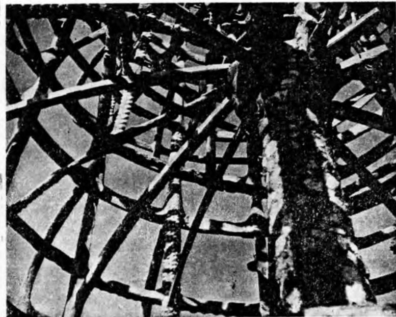
Fig. 3—Center column, rings and spokes of test tower
