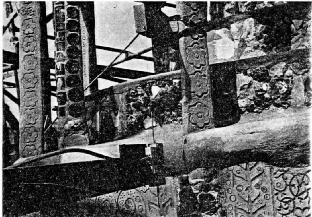
Fig. 10—Transducer installation at tower base (south side)
